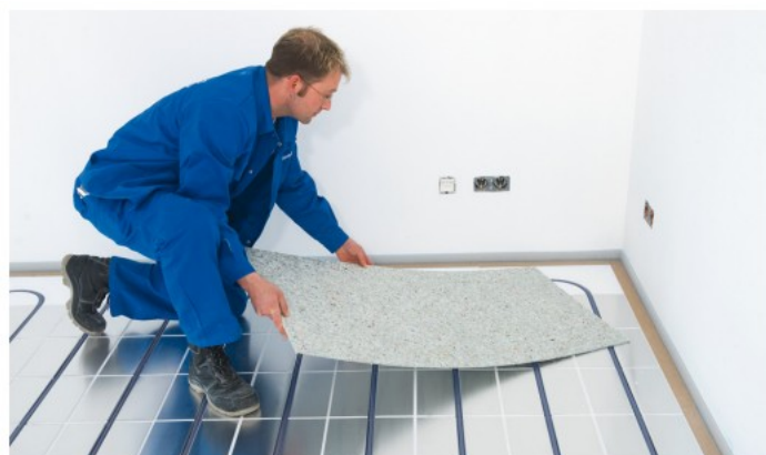
Fig. 1: Before applying adhesive, lay Strongboard in staggered pattern (see 3) onto the evenly laid heat panels.
