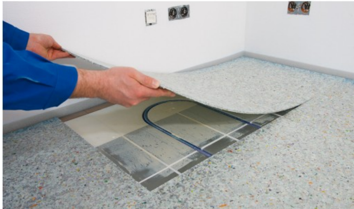
Fig. 7: Allow the adhesive (e.g. Ecofix by Mapei) to evaporate for 10 mins before continuing to lay the panels.
