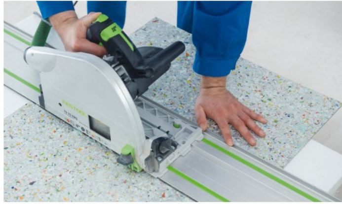
Fig. 2: Cut Strongboard with circular saw (universal blade). Use off-cuts at beginning of next row.
