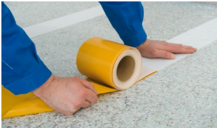
Fig. 8: Tape up all butt joints with 140 mm joining tape.
