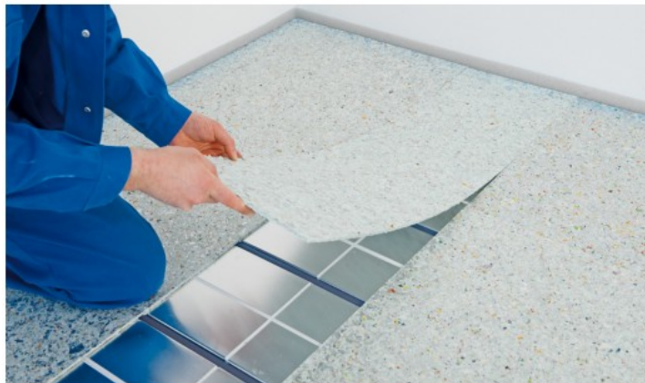
Fig. 4: Panels cut length-wise should be laid in the pen-ultimate rows and care should be taken to keep the staggered pattern.
