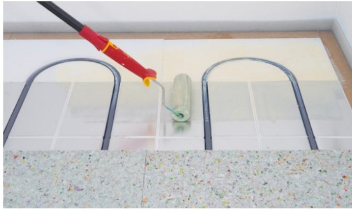
Fig. 6: Always use an adhesive to fix Strongboard to the heat panels.
