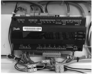
Picture 4: Temporary wiring
