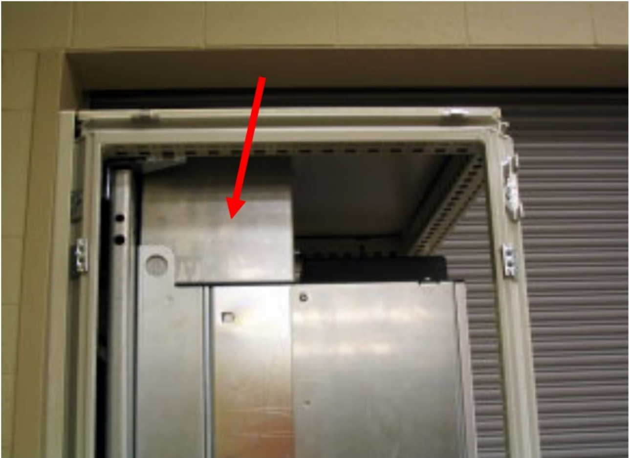
Photo 8. Top duct work and enclosure top installed.
