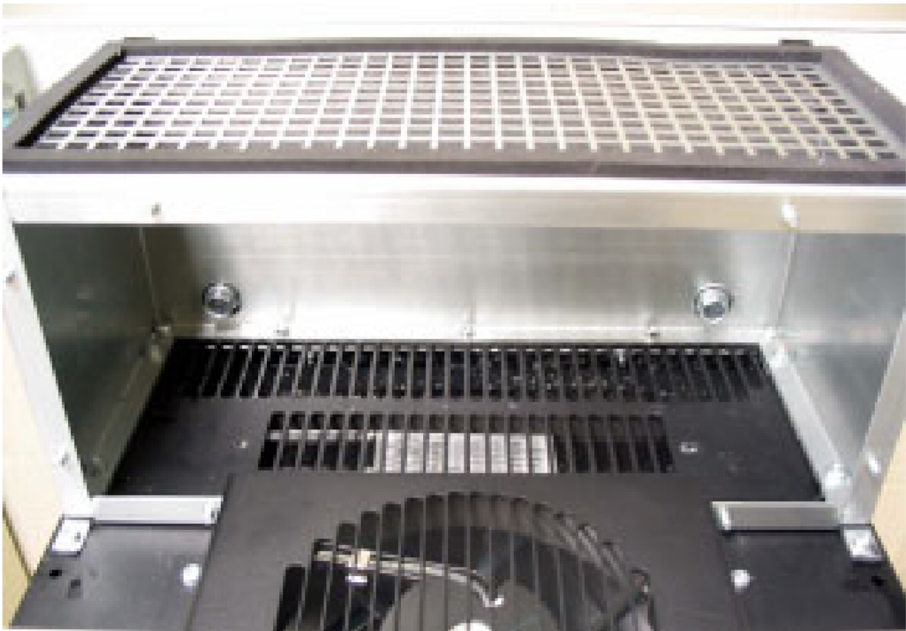
Photo 14. Top duct installed.
