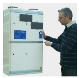
3. Remove the front foam panel to get access to the parts inside the unit.
