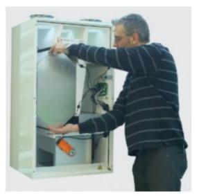
5. The heat exchanger can now be lifted/pulled carefully out of the core.
