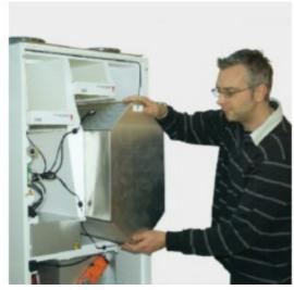
6. Pour a mild solution of regular dishwashing soap through the four open sides of the heat exchanger. Let it soak for 5-10 minutes before rinsing under running water. Dry the exterior of the heat exchanger, and gently slide the heat exchanger back into the unit.
