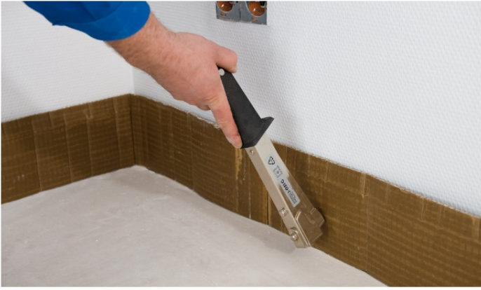
Fig. 2: Attach SpeedUp Eco perimeter insulation on the wall. Avoid overlapping the ends. 1
