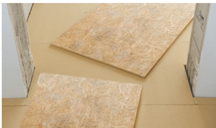
Fig. 10: Protect insulation from frequent pedestrian traffic to avoid damage.
