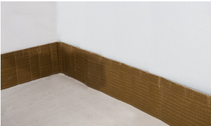
Fig. 3: Fold perimeter insulation to fit into corners.
