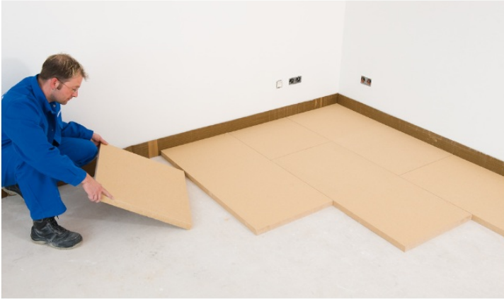
Fig. 6: Butt panels tightly to one another. Make sure the panels are level.
