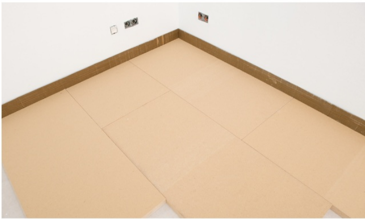
Fig. 7: Always cross-lay the second layer of insulation panels. The final layer of insulation must be cross-layed to the SpeedUp heat panels.
