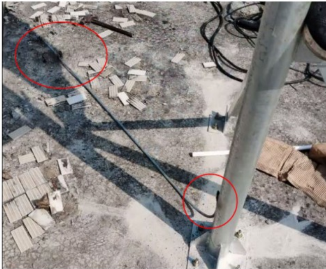
No lightning rod installed
