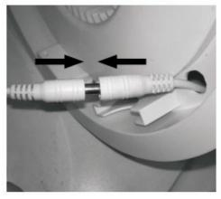
5. Push the LED cable connector back through the hole so the connectors are hidden in the ceiling cavity. (See diag. 4)
