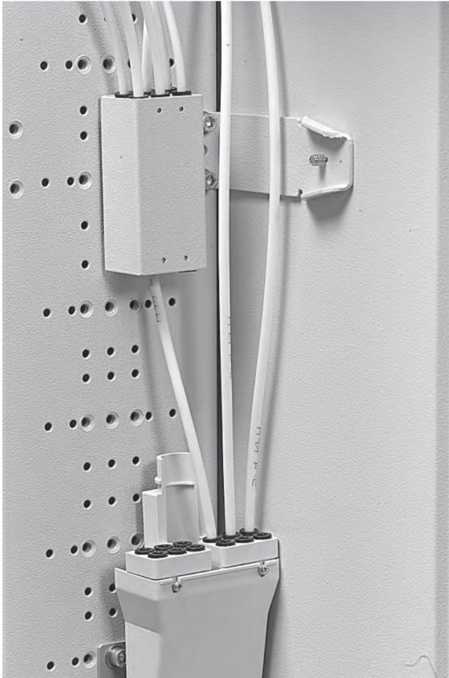
The tube divider FIST-GR-TD-5mm can be mounted in the rack. Install as shown. IN: maximum 6 tubes. OUT: maximum 6 tubes
