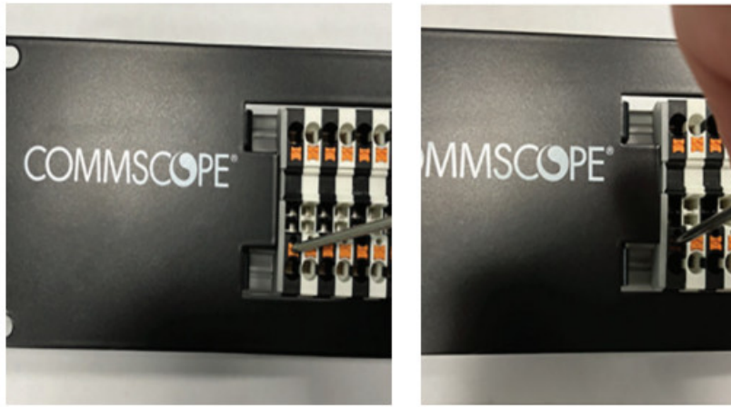
Figure 5. Releasing the Clamp
