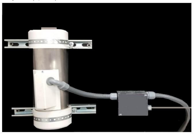
Shown above: V18 mounted on a painted plywood board with Uni-struts. Or mount to other wood mounting, not metal. Flow must enter from the bottom, plastic cover should be closer to the bottom as shown
