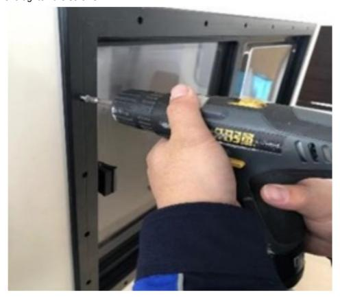
6. Once the window installation is complete, the optional blackout system can be installed if required. Depending on the installation situation and the existing wall thickness, an additional wooden frame may be required for mounting the blackout system. This must be manufactured individually and by the customer. At the four outer corners of the frame are the holes for the screw connection. Fasten the blackout system with the supplied
