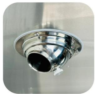
9. Using the included hex wrench begin tightening the screws in a clockwise direction while holding the vent agains the ceiling. Stop as soon as you feel slight pressure. Continue to the next screw. Do a 2nd pass on all the screws to finish tightening. The assembly should be fully flush with the ceiling.
