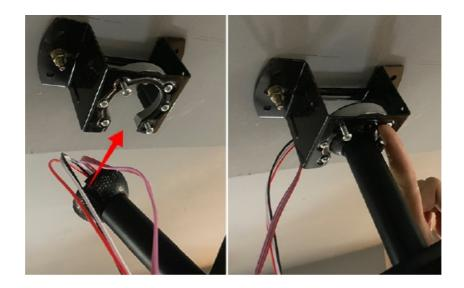
Connect the wires on the controller (1) with the ceiling fan and your L & N line.
