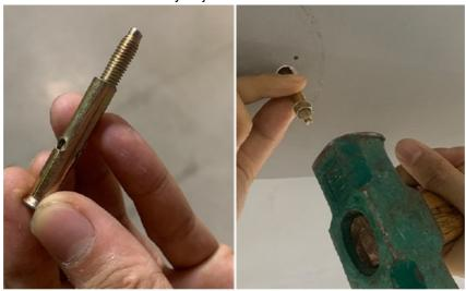
Assemble and tighten the hanging bracket.
