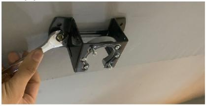
Put the ceiling fan which well assembled on the hanging bracket, gentely rotate the lever to make it perfect fixed on the bracket.
