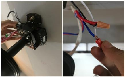
Sort the wires and push the big hanging cup to the top to cover all the wires and parts. Gently rotate and tighten the cup and lever.
