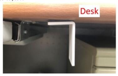
Step 4 Stick the sensor with another 3M VHB double-sided tape (size not bigger than  $30 \times 30$  mm, or we have this size of tape in stock!)
