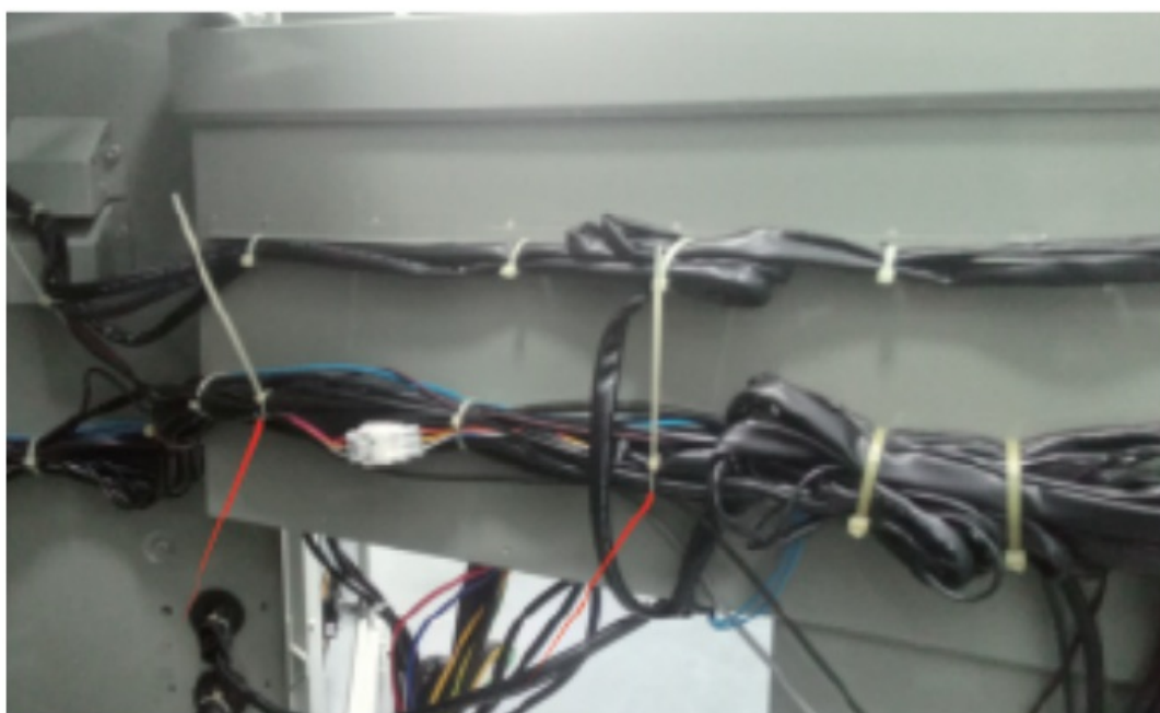
Figure 9. Cross, fixed, locking and binding wire
