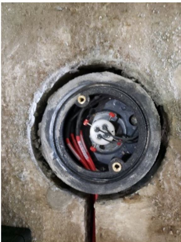
Figure 17: Sensor cables tucked in, roadbox cover reinstalled
