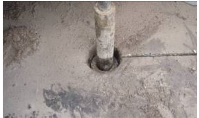
Figure 8: Wooden doughnut being used to guide the split spoon through the center of the corehole
