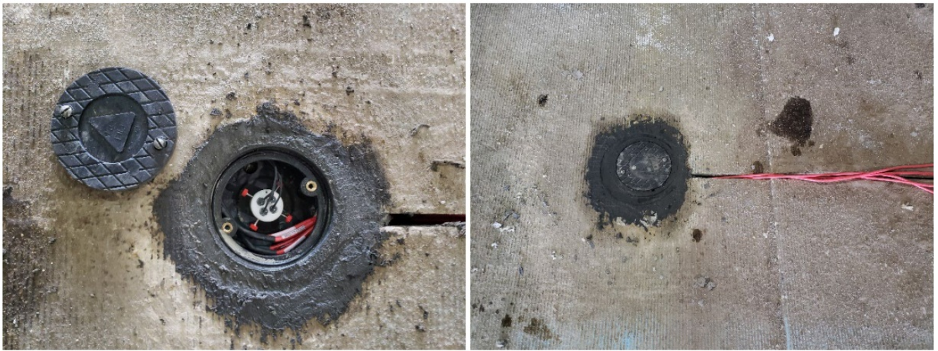
Figure 18: Annular space surrounding the roadbox filled with dyed Quikcrete ®
