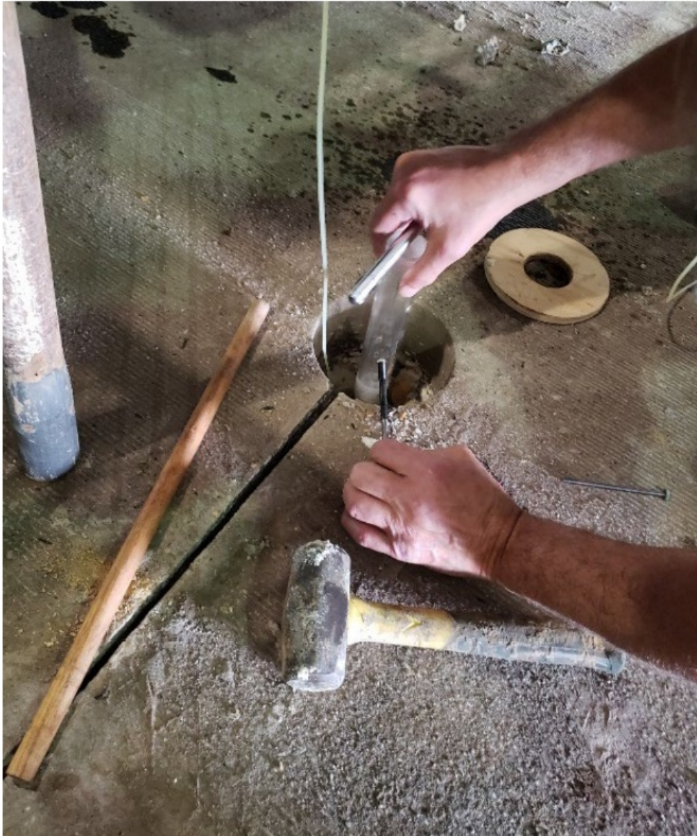
Figure 9: Connecting rod being inserted into the setting tube, in preparation for setting the hydraulic anchor d. Once the connecting rod is resting against the road surface, and the stop nut is against the top of the head unit, attach the free end of the hydraulic tubing to the hydraulic hand pump from the installation kit. Begin filling the bladder of the anchor.
