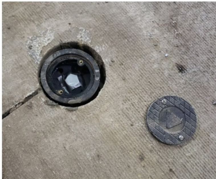
Figure 12: Roadbox screwed onto the head unit, protective tape replaced over measurement holes
