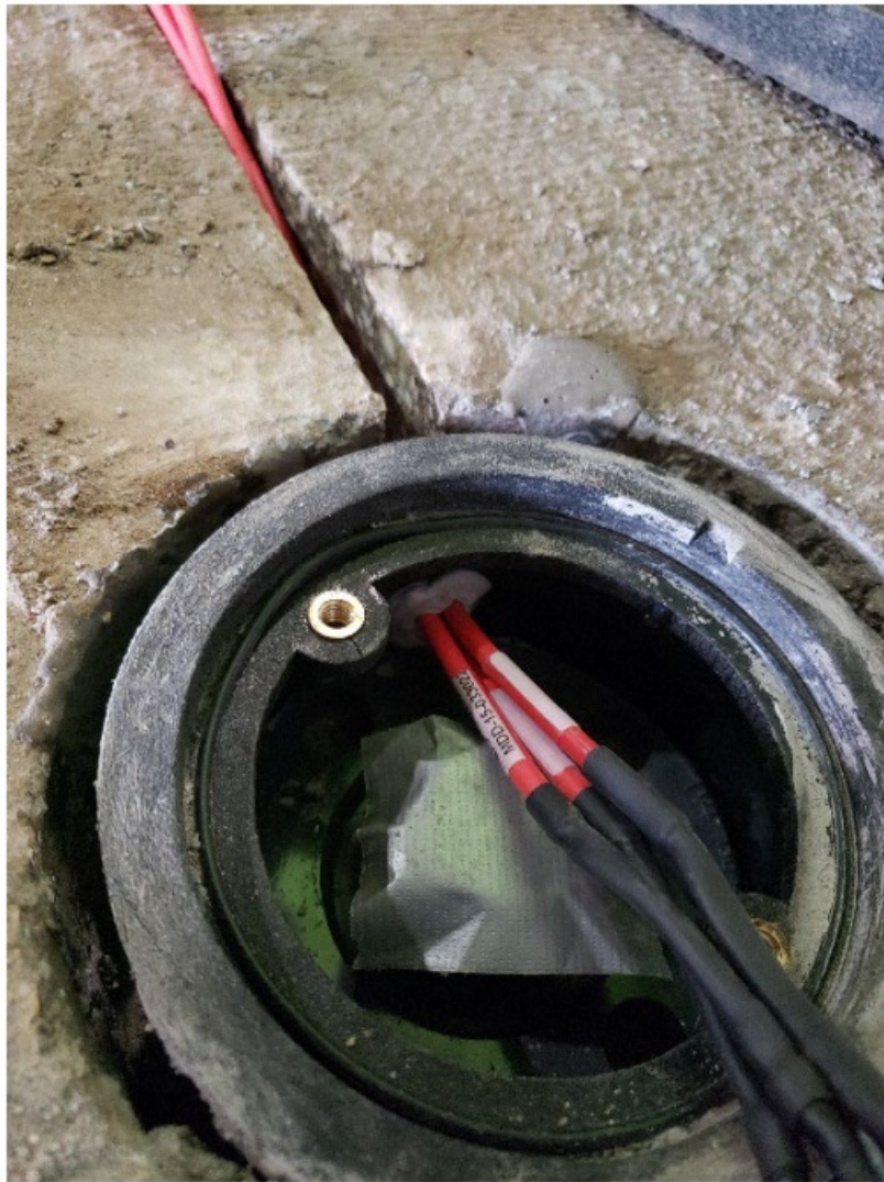
Figure 15: Butyl rubber stopper placed into the cable exit, while also surrounding each sensor cable
