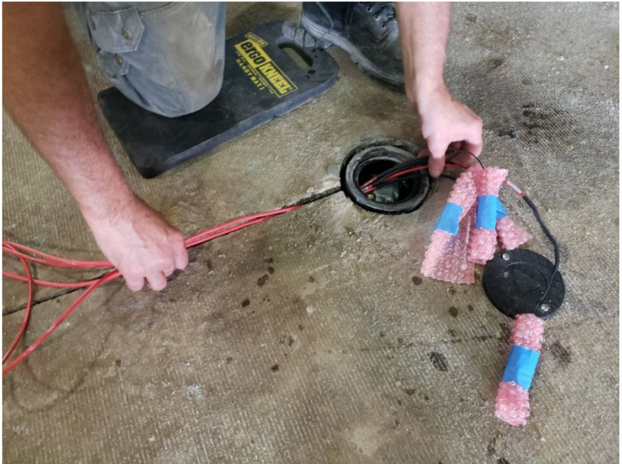
Figure 14: Sensor cables fed through the cable exit and along the trench
