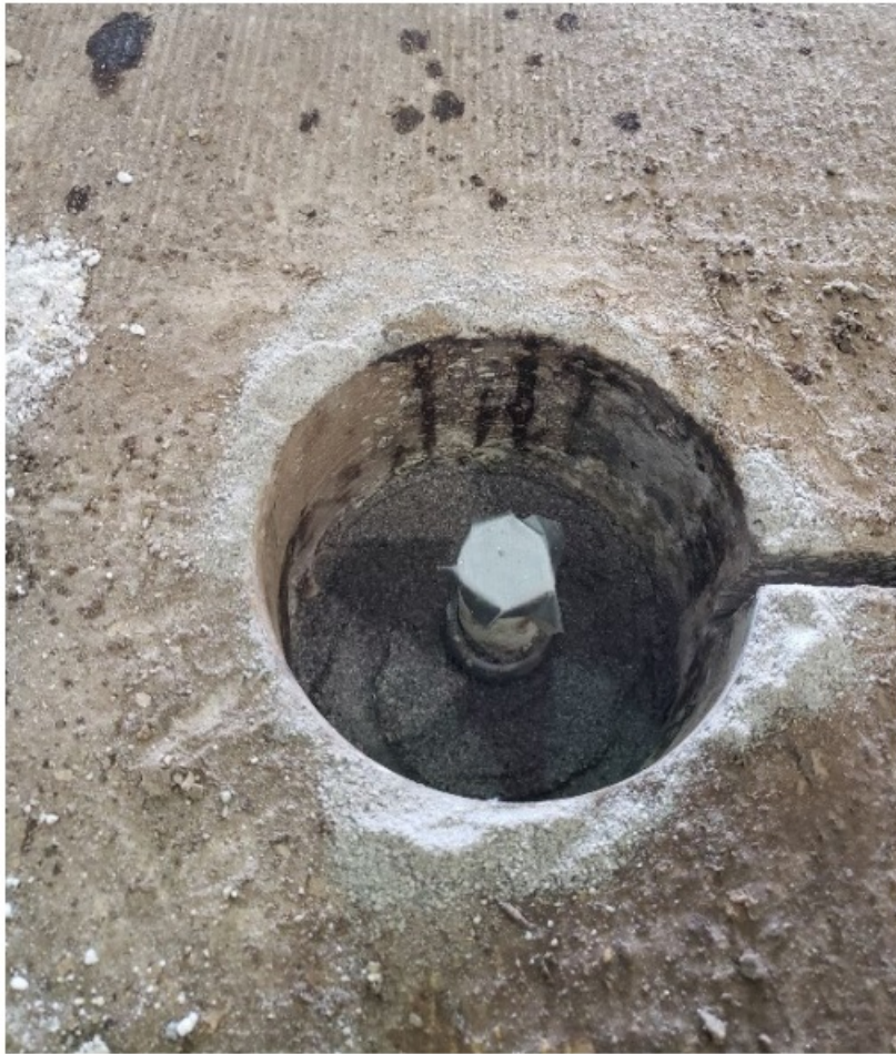
Figure 11: Head unit covered and layer material placed around the top of the duct hose
