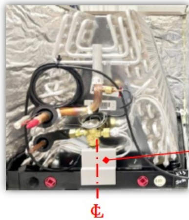
VERTICAL/UPFLOW CONFIGURATION (uncased/cased)
