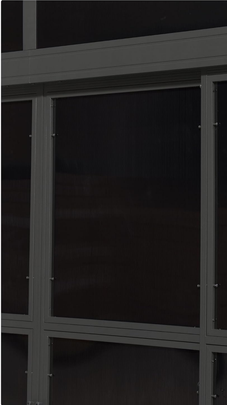
Figure 5.1: PC panels for weather protection and mesh for ventilation.
