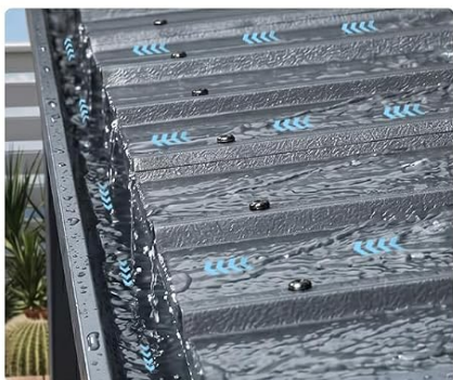
Gutter collects water along the front edge
