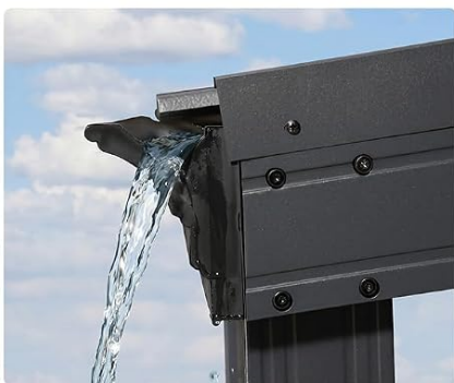
Downspout directs water to ground level
