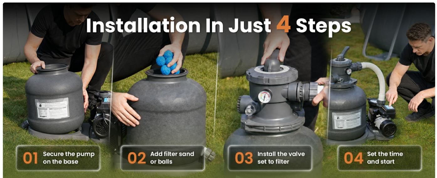
Image: A visual guide demonstrating the four key steps for installing the sand filter pump.
