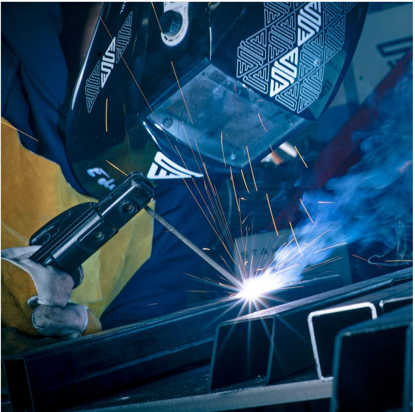
Image 7: MMA welding on metal profiles, showcasing the process.
