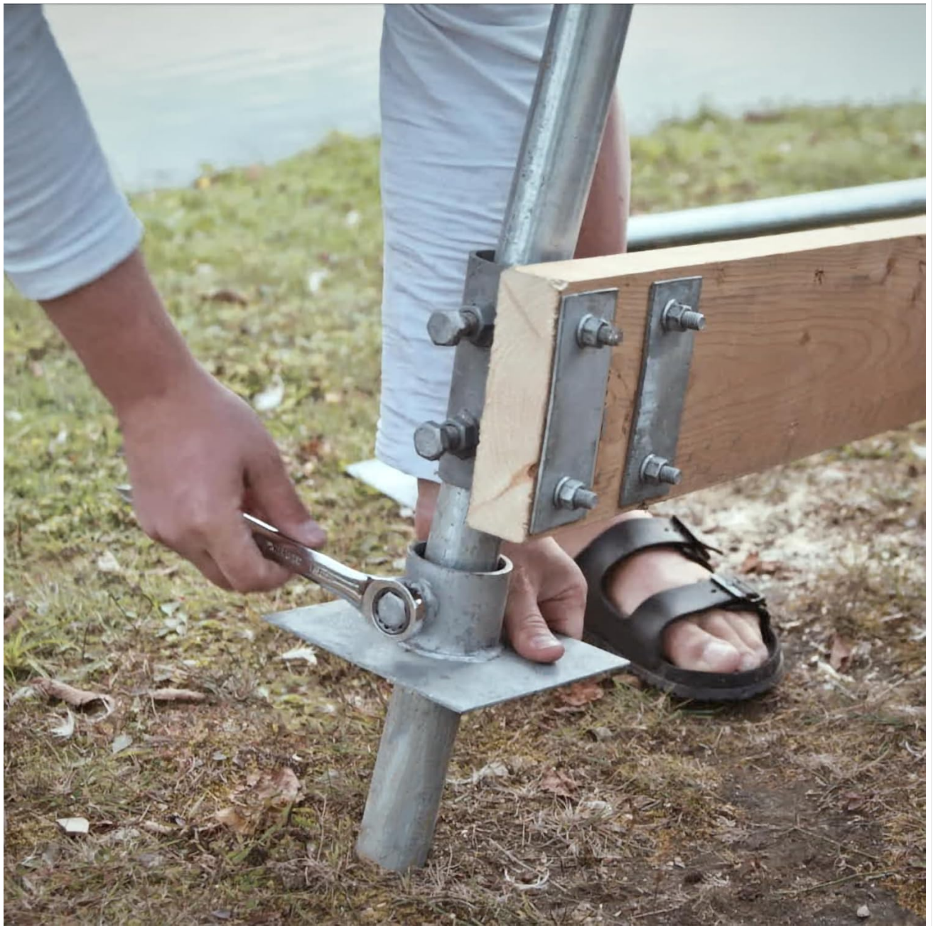
Image: Adjustment of the ramp's height and stability using the provided posts and base plates.
