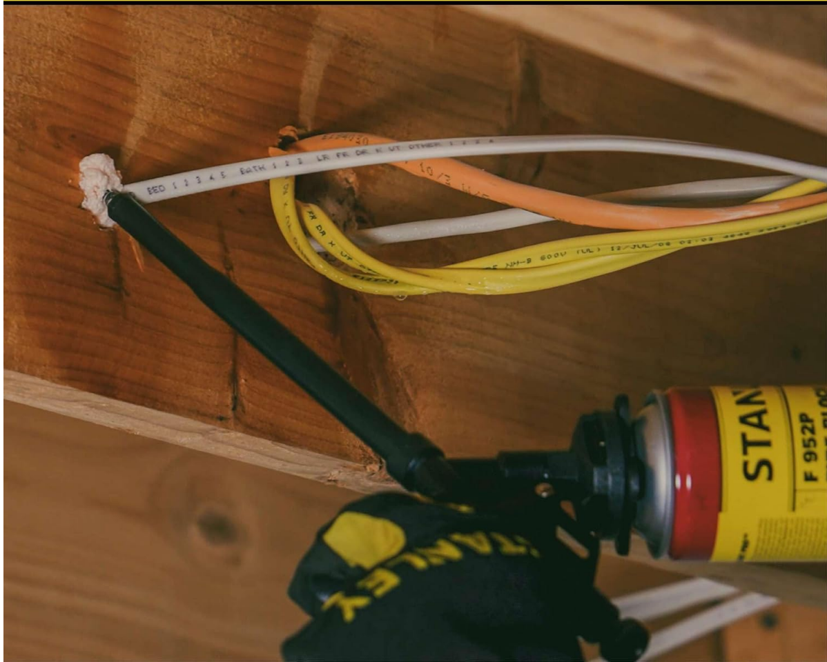
Image: Insulating pipes and HVAC ducts for energy efficiency.
