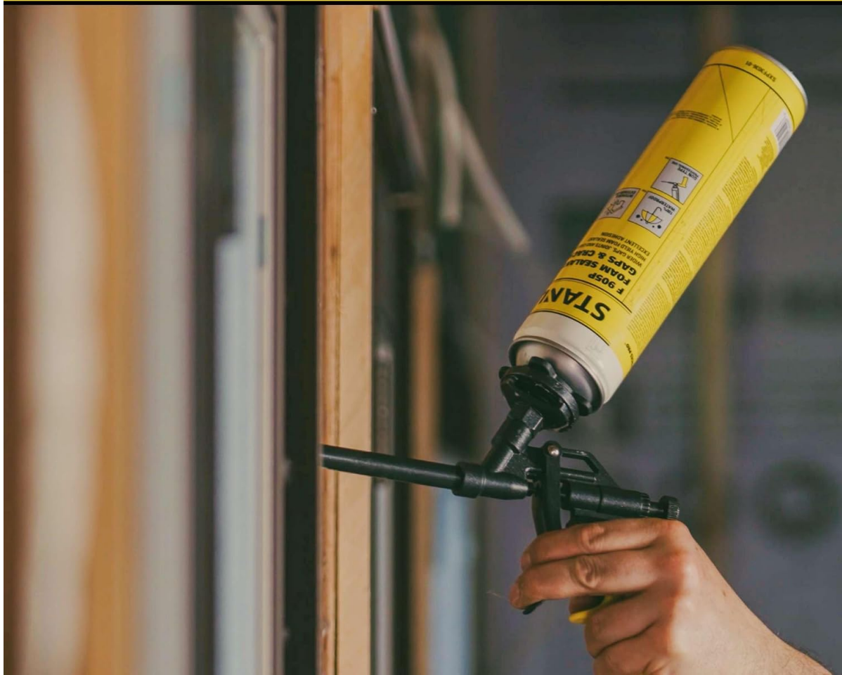
Image: Filling cracks in a wall for improved insulation.
