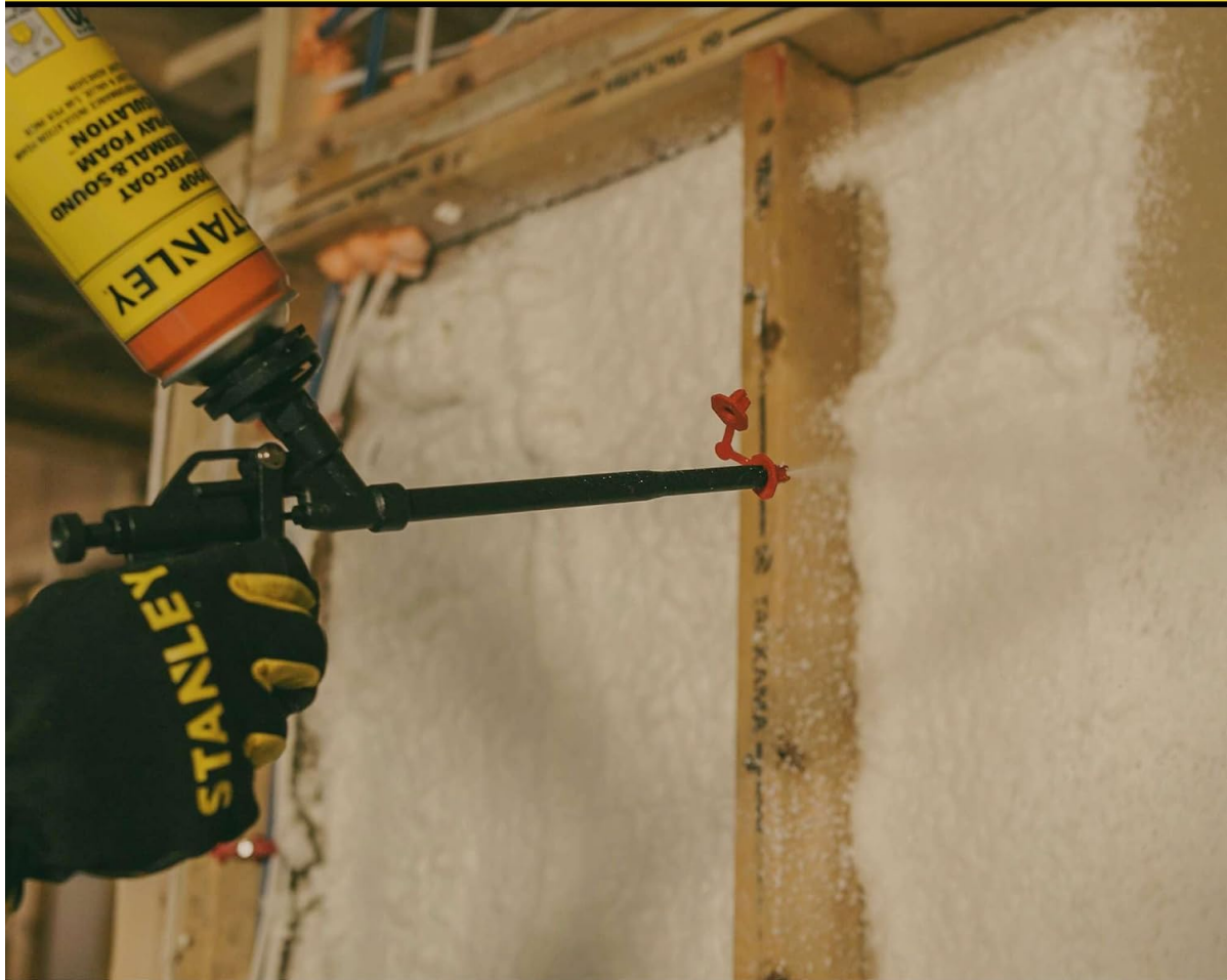
Image: Application of foam for soundproofing and thermal insulation.
