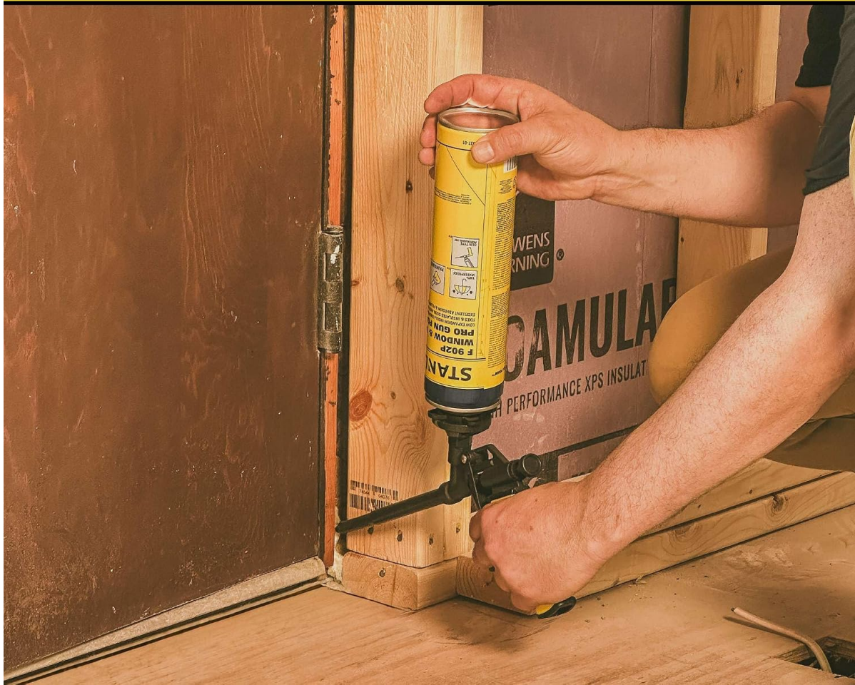
Image: Sealing gaps around a window frame using the foam gun.
