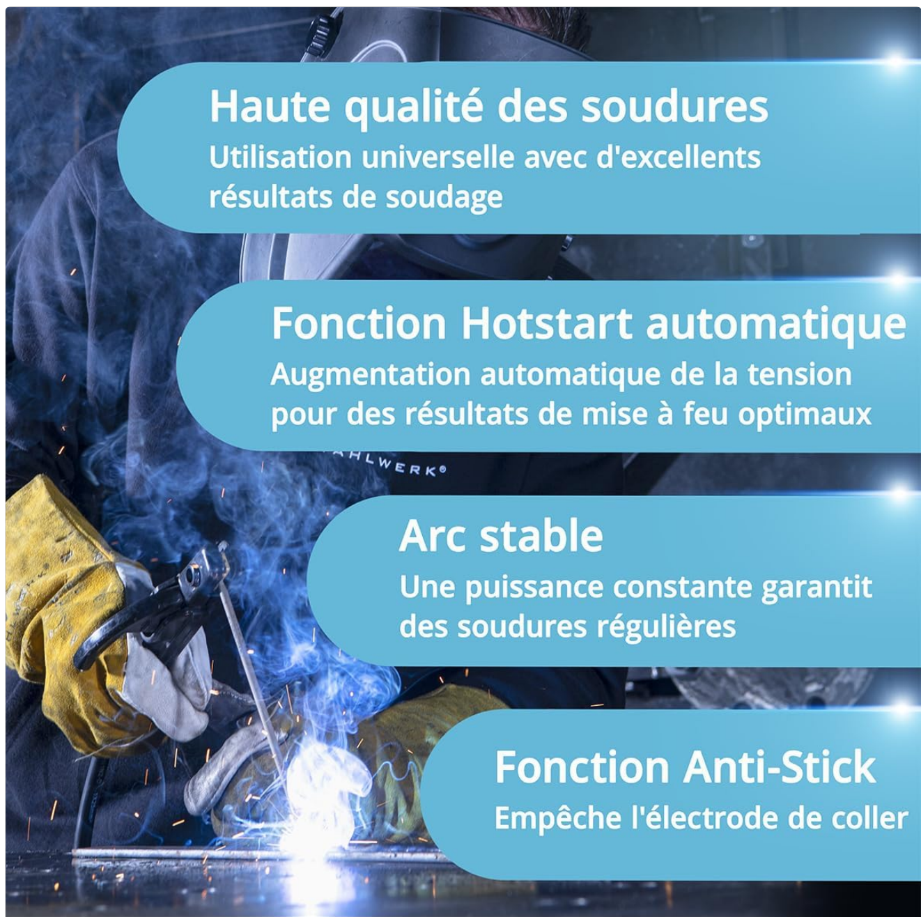
Figure 5: Welding in progress, demonstrating the stable arc and benefits of Hotstart and Anti-Stick functions.
