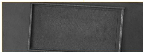
ONE-WAY VENT TO PREVENT CONDENSATION
