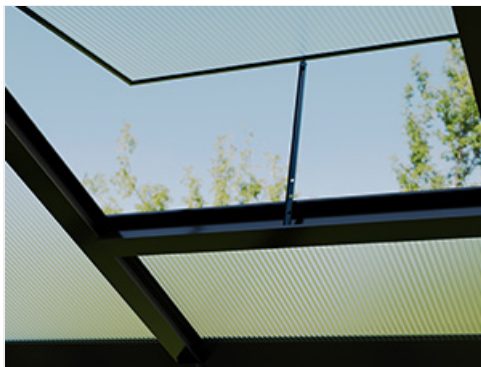
Figure 4: Height-Adjustable Windows. This image shows the mechanism for adjusting the roof vent to control ventilation.
