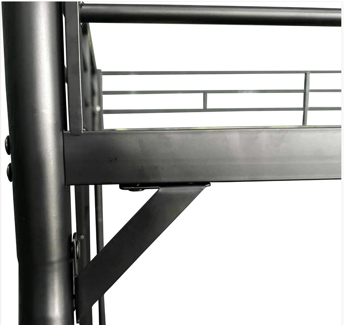
Image: Close-up of a frame joint, showing connection detail.
