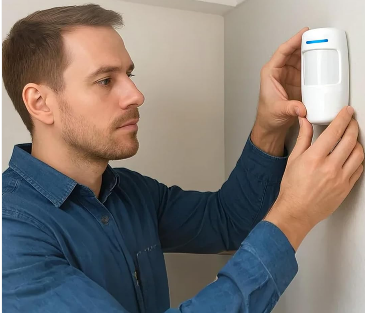
Figure 4.3: Motion Sensor installation.
