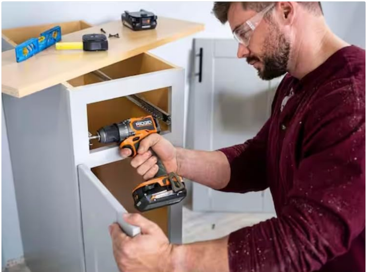
Figure 7: Installing cabinet hardware with the drill/driver.
