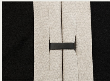
Screw clip fixing
