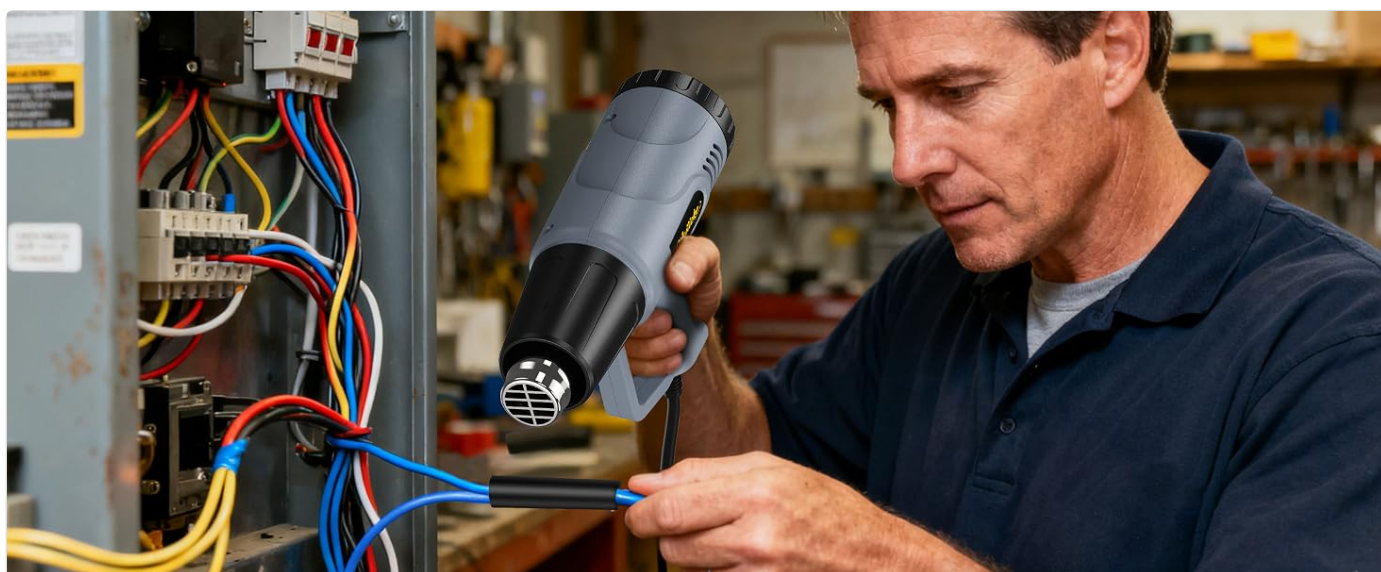
Figure 6: Applying heat shrink tubing with the heat gun.
