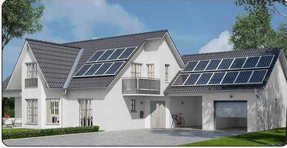
Solar Home System
