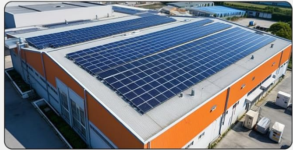
Solar Power Plant System
