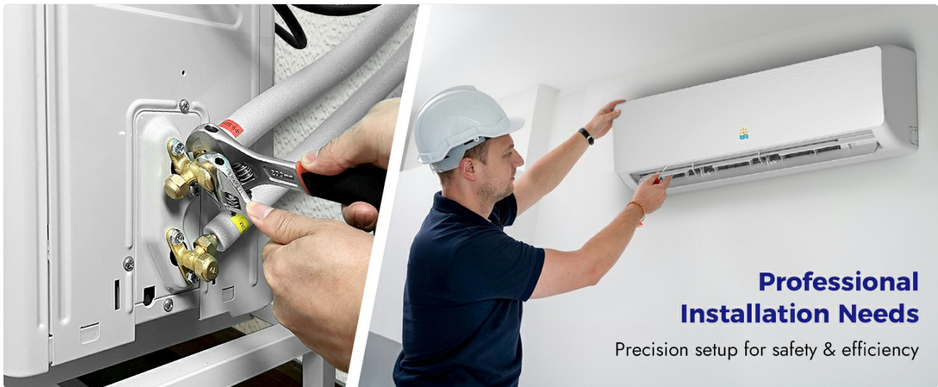
Image 4.1: Professional installation of indoor and outdoor units.
