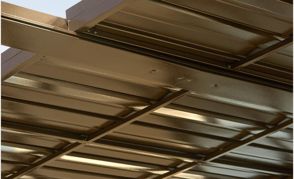
Image 6.1: A detailed view of the galvanized steel roof construction.
