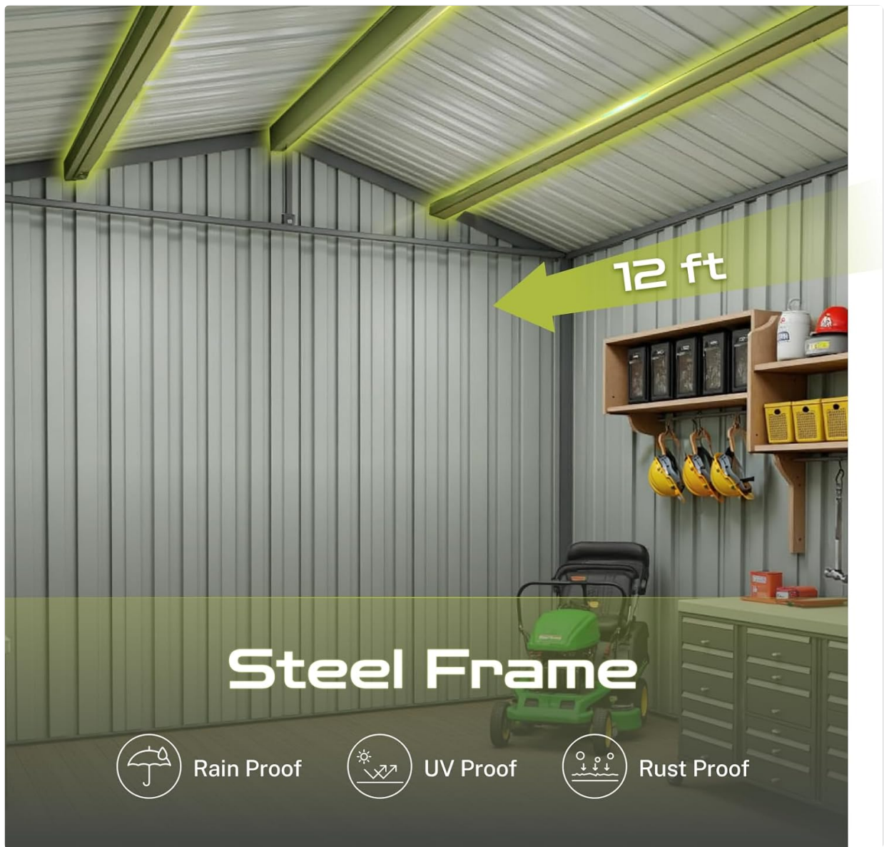
Figure 2: Interior view showing the robust steel frame construction.
