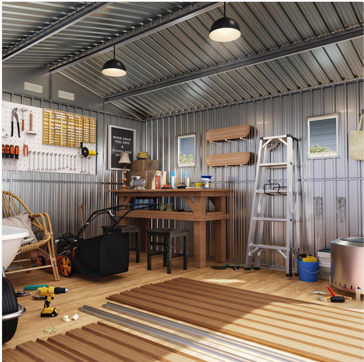
Image: An interior view of the shed during assembly, showing various tools, partially assembled wood-grain panels, and a ladder, indicating the ongoing construction process.
