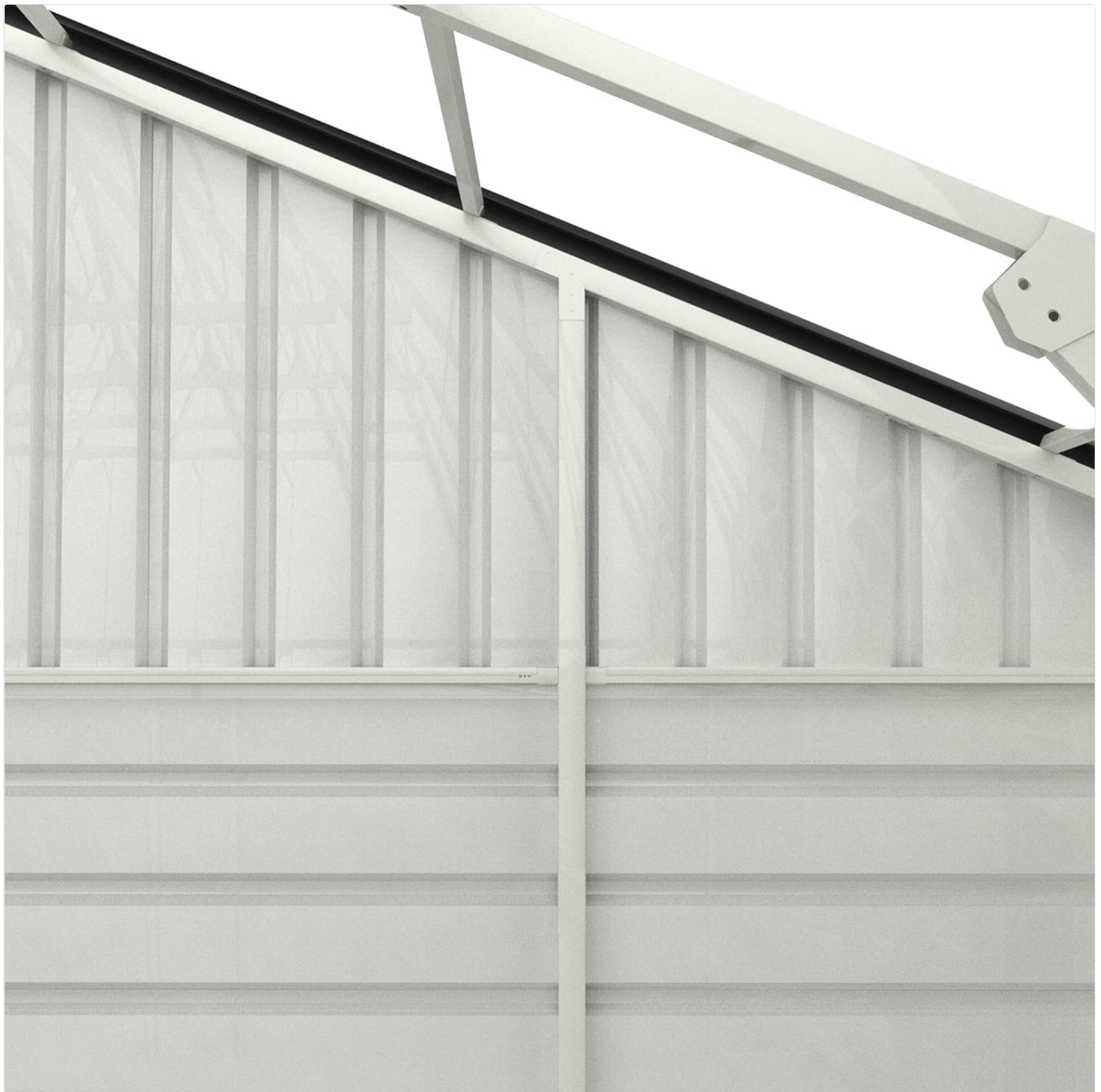
Image: A detailed close-up of the shed's interior, focusing on the connection point between the roof paneling and the top of the wall. This highlights the corrugated metal design and the structural beam running along the roofline.
