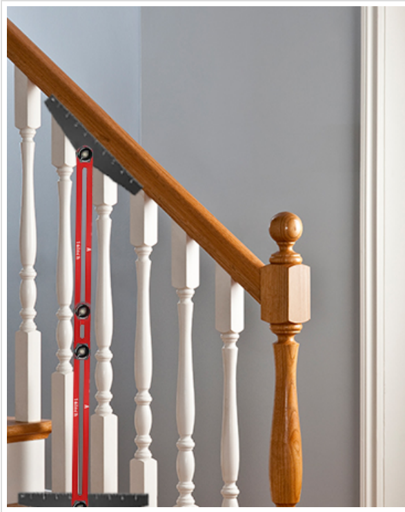
Figure 6: Marking the outline using the adjusted template.
