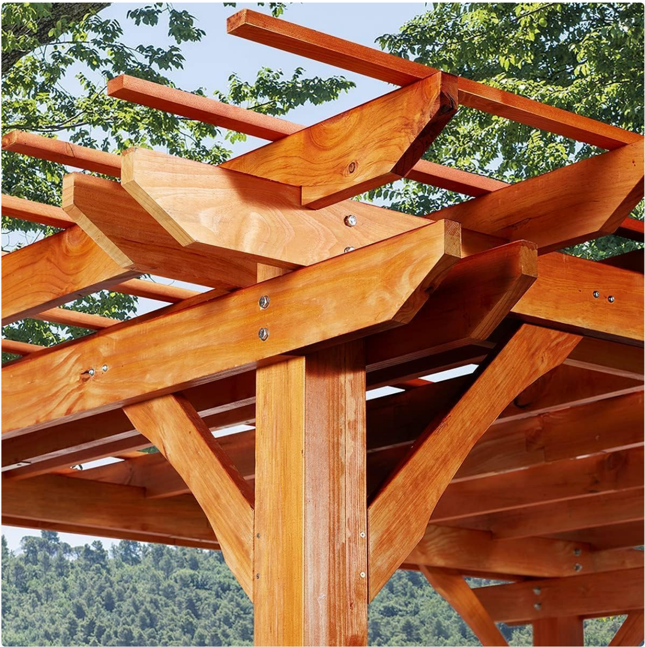
Image 4.1: Detail of the robust roof structure and support beams.
