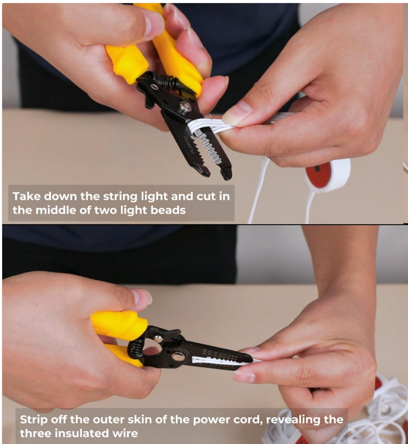
Figure 4: Cutting and stripping wires. Use appropriate tools to expose the internal wires for connection.
