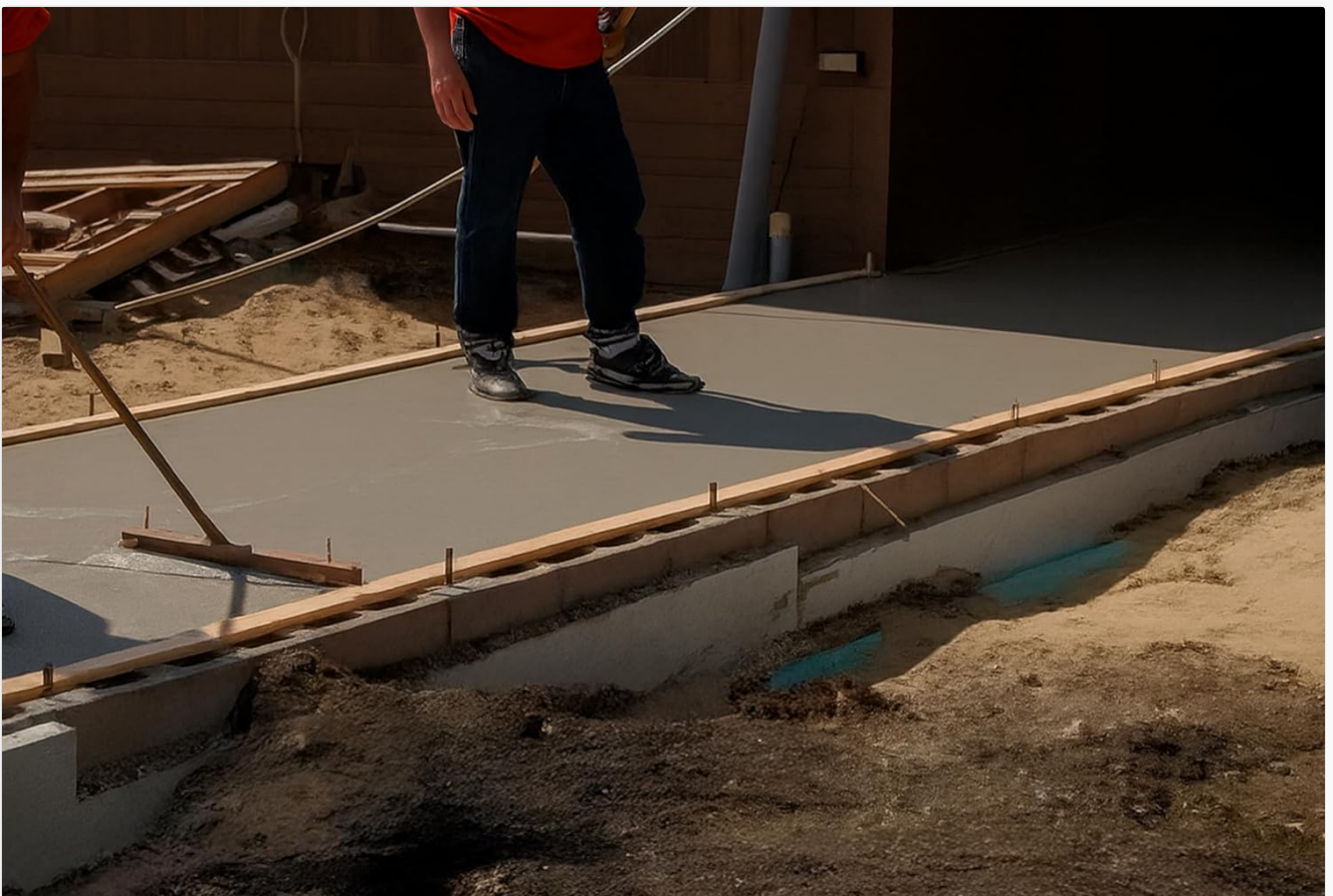
Figure 5: Finished leveled surface. This image shows a large, smooth, and evenly leveled concrete surface after the application of Ardex K 301.
