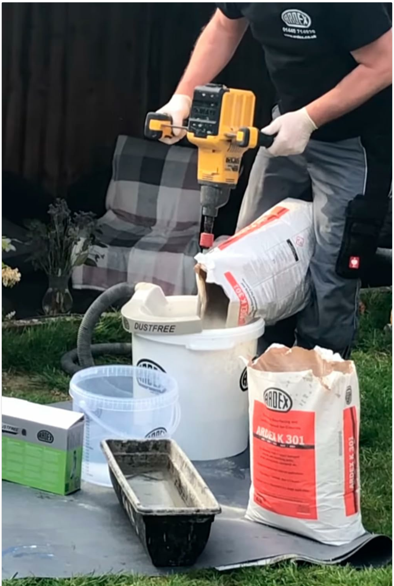
Figure 2: Mixing Ardex K 301. A person is shown mixing the Ardex K 301 powder with water in a bucket using a heavy-duty drill and mixing paddle.
