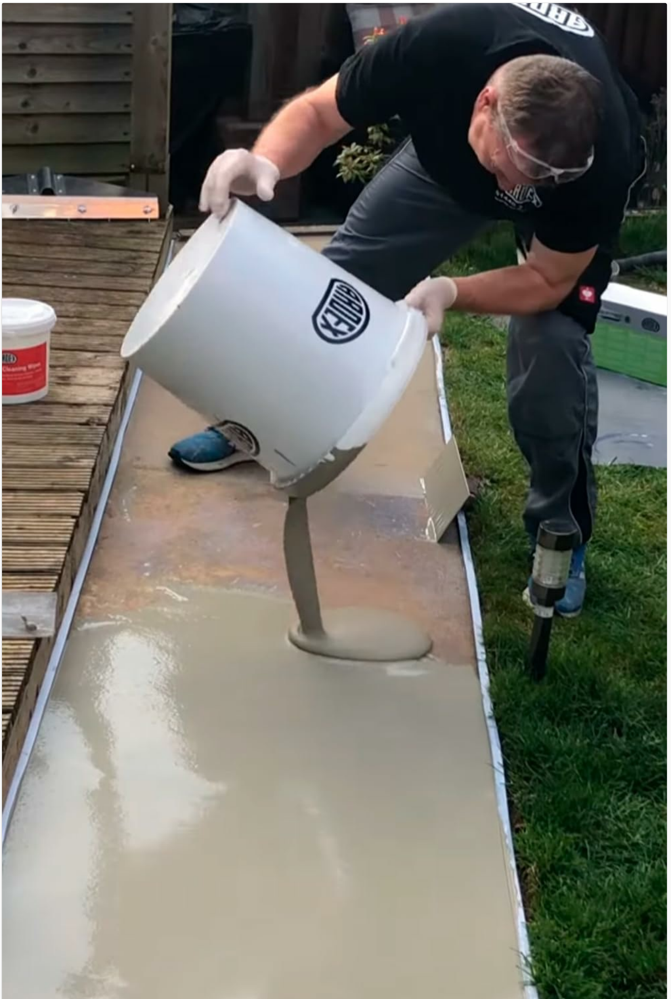
Figure 3: Pouring Ardex K 301. A person is pouring the mixed self-leveling concrete from a bucket onto a prepared outdoor surface.
