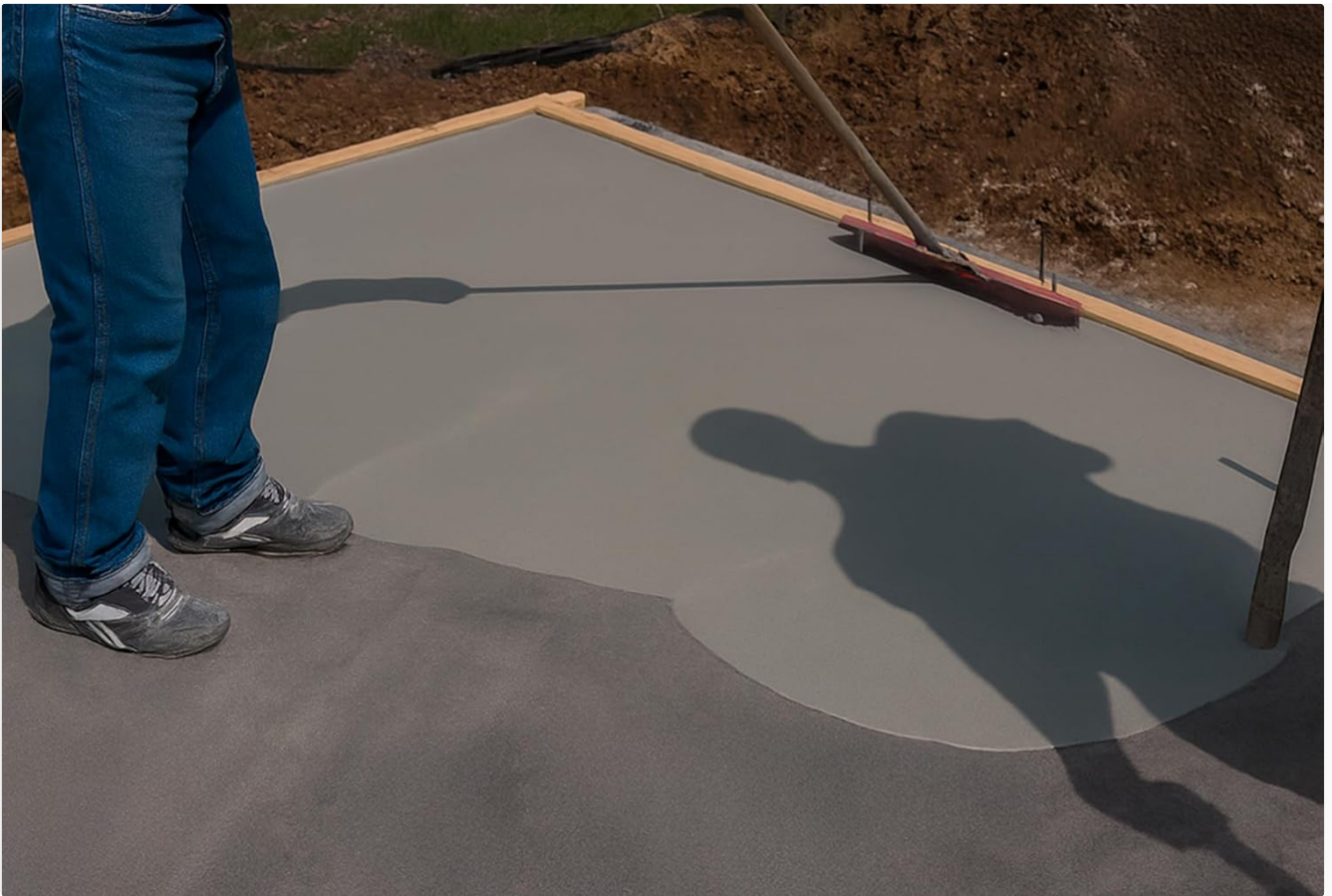
Figure 4: Spreading Ardex K 301. A person is using a long-handled gauge rake to evenly spread the freshly poured self-leveling concrete across the surface.
