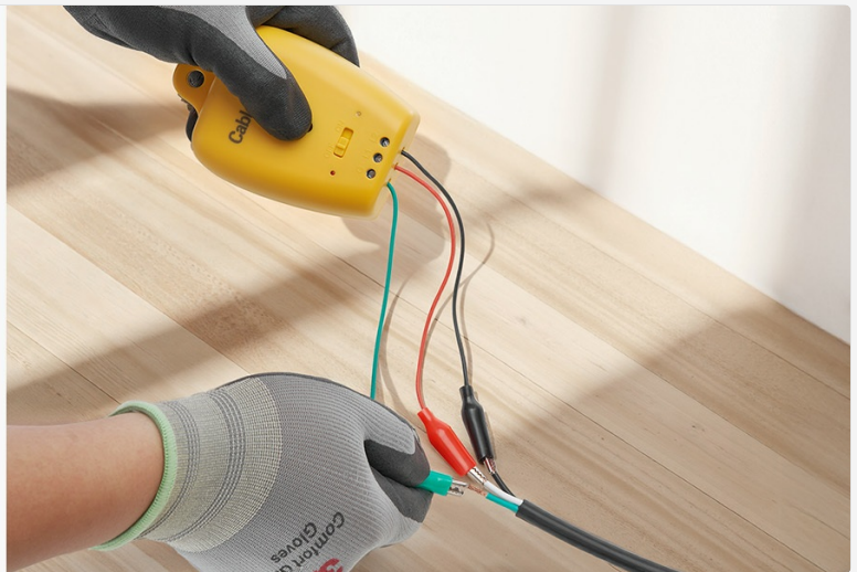
Image 4.3: The installation monitor connected to the heating cable for a pre-layout damage check, ensuring the cable is intact before installation.
