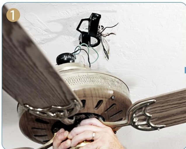
Disconnect the ceiling fan wiring
