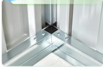
Image 6.1: Features contributing to shed stability, security, and weather protection.
