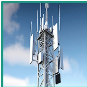
Image: Testing telecommunication towers.
