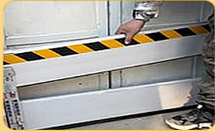
4. Install the baffle plate
