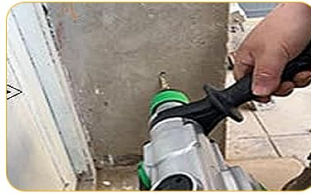
2. Drill the holes at the marked positions
