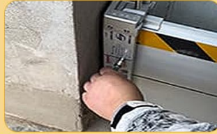
5. Tighten the screws on the side of the column
