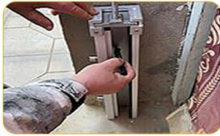
1. Mark the hole punching position with a marker pen
