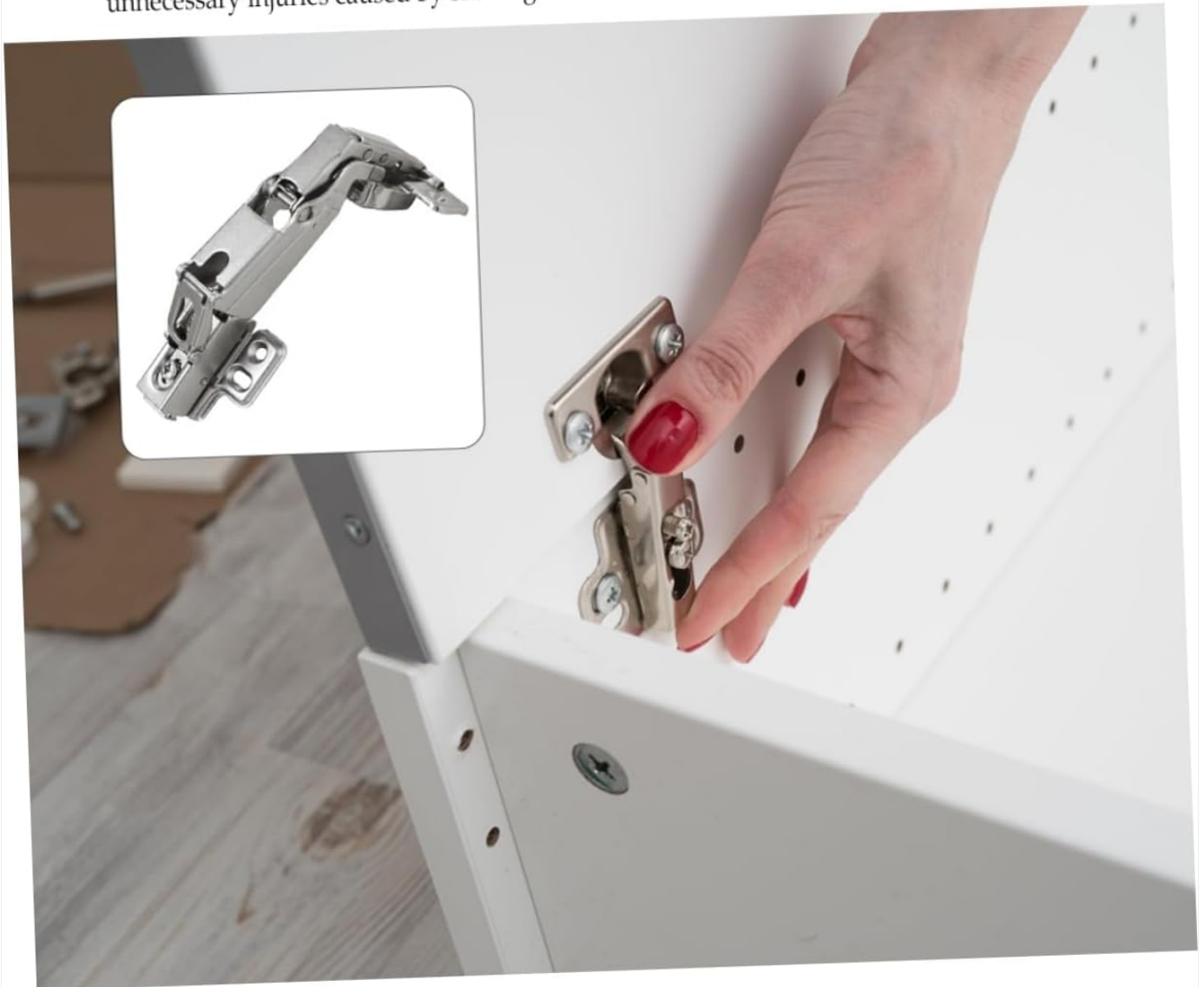
Image: Hinge being installed on a cabinet. This image shows a hand securing the hinge to the cabinet frame, demonstrating a key step in the installation process.
