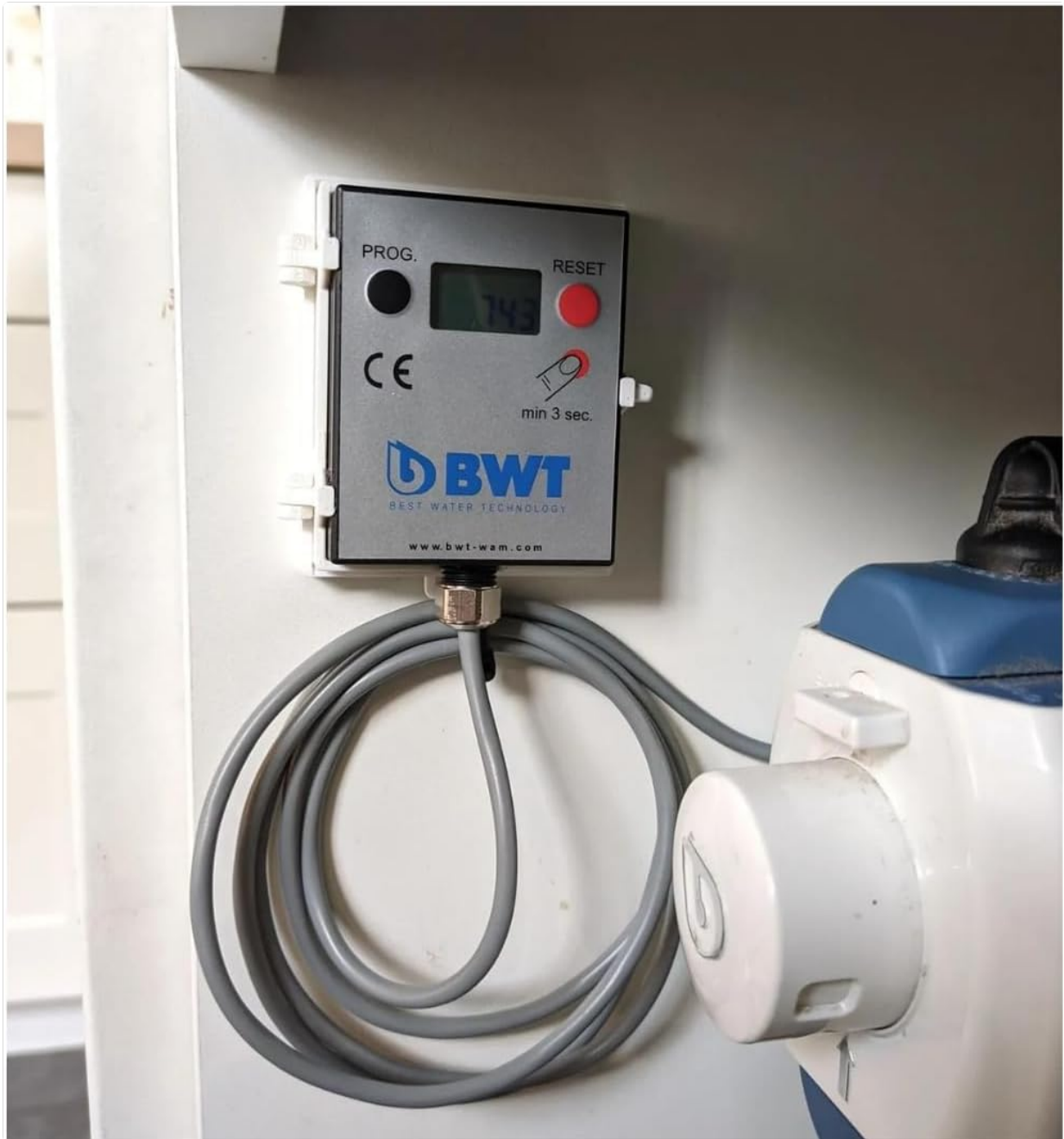
Image 5.1: Example installation of the Aquameter display unit.
