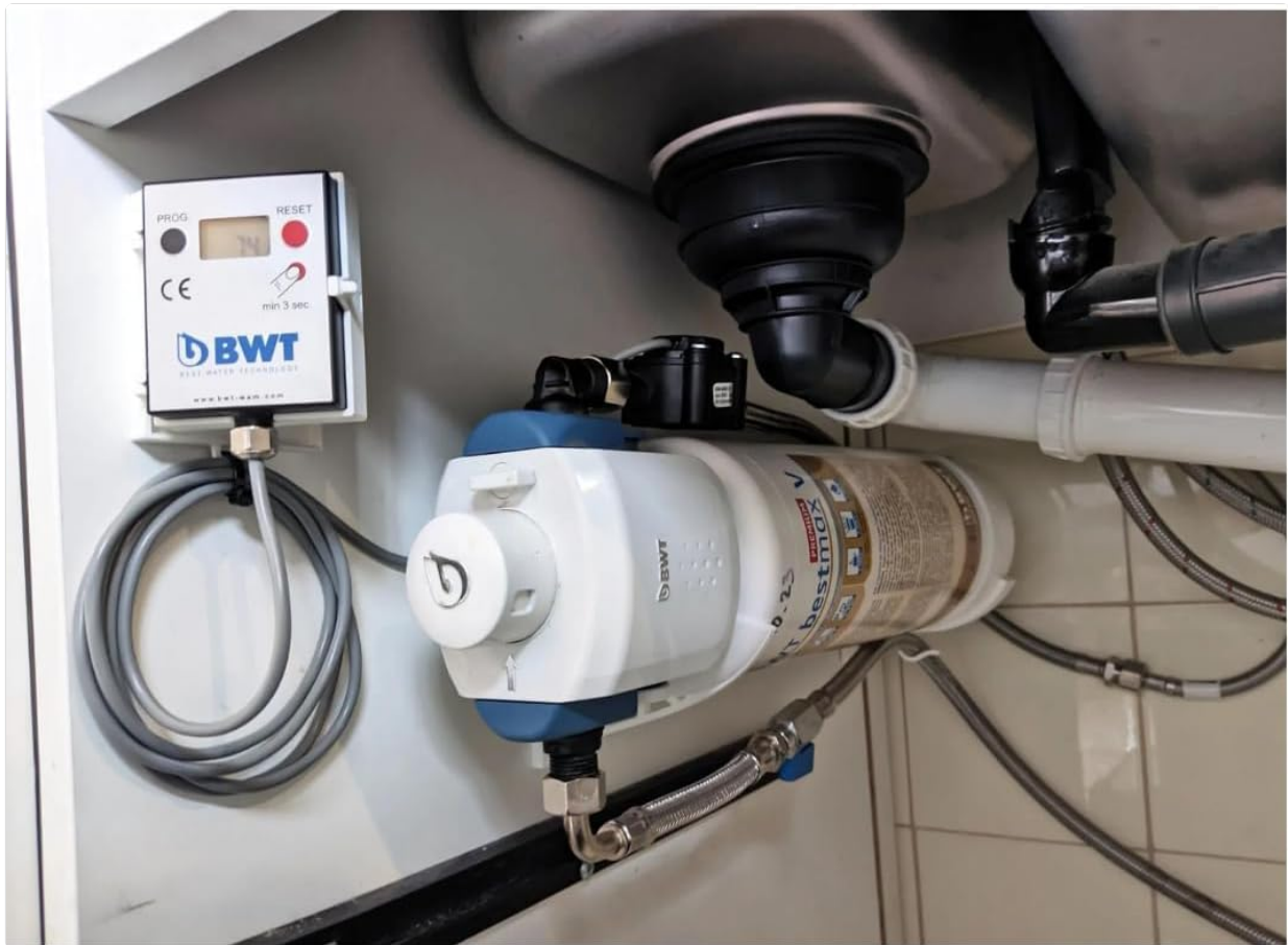
Image 5.2: Aquameter and filter installed in an under-sink setup.
