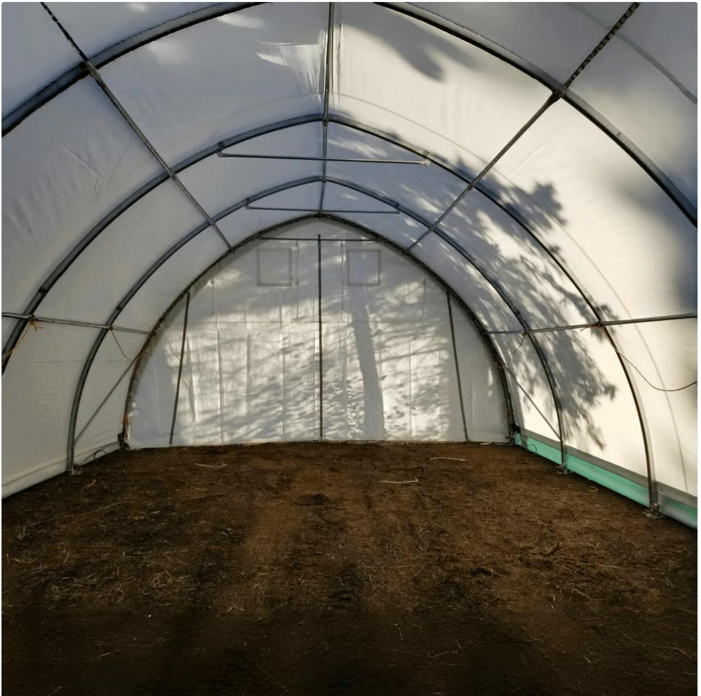
Image 5.1: Interior view of the storage shelter, showing the truss frame structure and spacious area.
