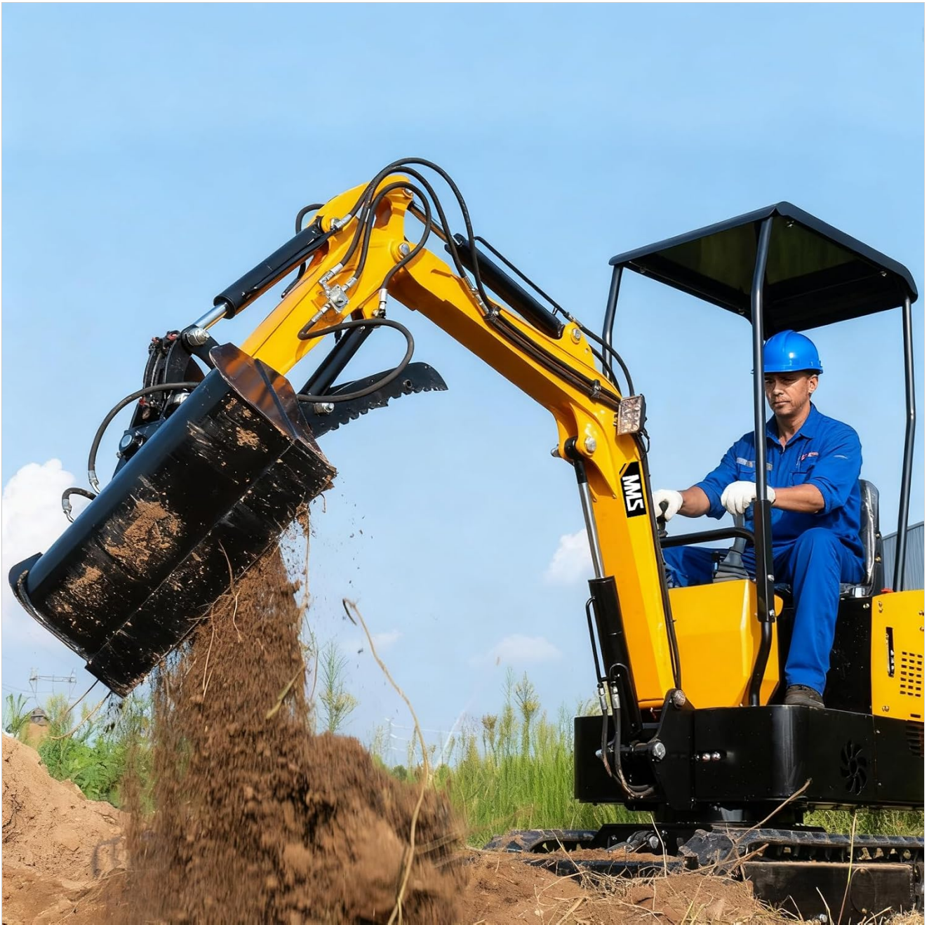
Figure 3: An MMS mini excavator utilizing the tilting bucket attachment to move soil. This image illustrates the bucket in action, demonstrating its capacity and the excavator's ability to perform earthmoving tasks.
